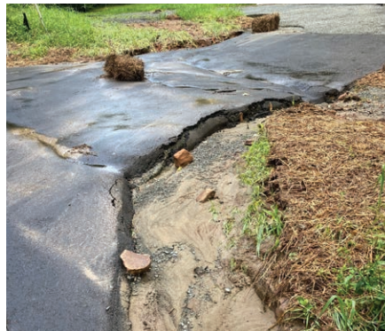
Damage from flood waters at the new Tanager Hill parking area wiped out a bridge and eroded the new paved driveway.
